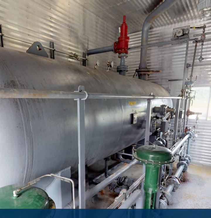
Ready to go! Sour rated but only ever operated in sweet service! This 60" x 300# separator built by ARGO Sales is their standard design/stock unit. It's a simple and effective unit: solid design, three province registration, 3 Phase Dressed 3, metering, fuel gas scrubber and a comprehensive end device package fully wired to JB's. Located close to Calgary for personal inspections and can be moved out anytime.
