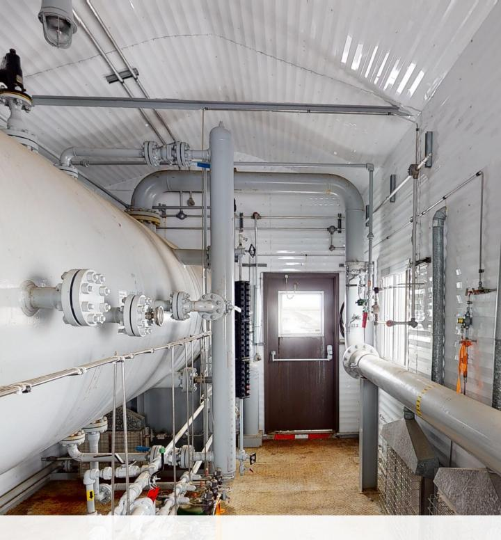
This separator is in great condition – built for sour and only ever used in sweet service. Commissioned in 2008, the vessel is currently setup for 2 phase service (water dump and panic dump), however all the connections and weir exist for it to have a 3rd phase added (1 week delivery and ~\$10,000). Full drawings, over 80 pictures, and more detailed information available upon request! Call us today!
