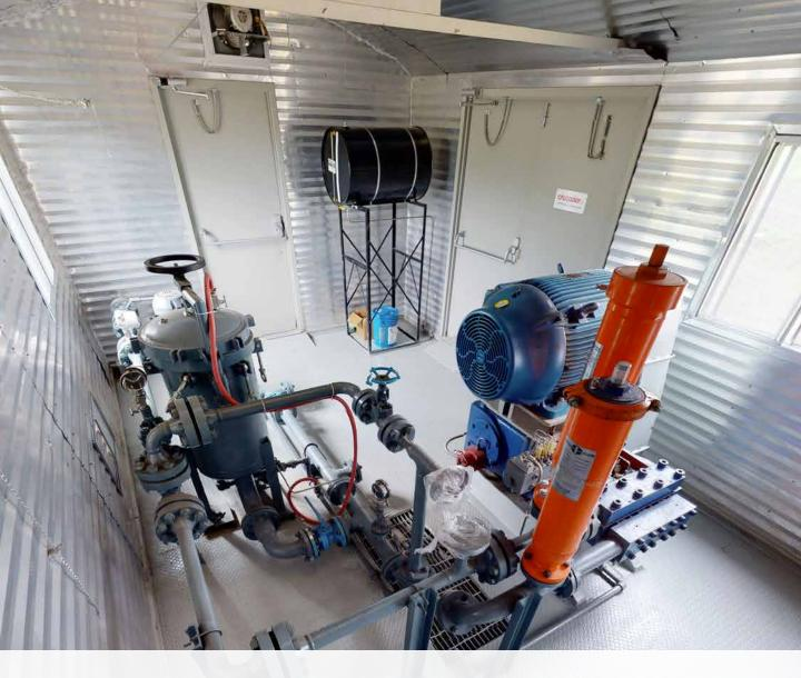
Up to 560m³/day or up to 3748psi discharge pressure – this full sour water injection / disposal package is sitting right now in Three Hills, AB and can go to work immediately after installing your choice of plungers! The Union TD-120 Pump is the only part that is in a reconditioned state, everything else is in unused/new condition. Fortunately, we did the pump work ourselves, so we offer a full 1 year warranty on it – the same that you would get if you bought a NEW pump from Union or National.
