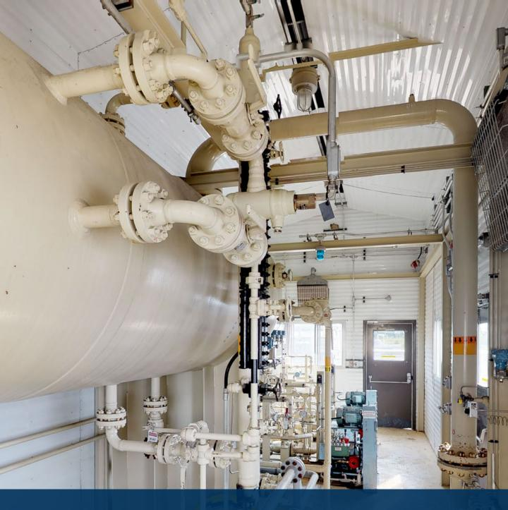
A clean, well appointed 48" separator package. Built by Presson in 2000, this unit was designed to pump condensate right off the bottom the vessel via dual Wheatley T255M triplex pumps w/ 1.25" plungers. Vessel is a 2 Phase design shut down & blocked in in 2013; opened, cleaned and installed a nitrogen blanket in July 2015. In addition, everything is fully wired to junction boxes c/w lights, fire loop, beacons, ESD, 120V start Catadynes, exhaust fans etc. Located by Rocky Mountain House.
