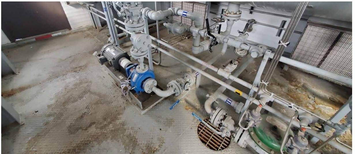
The Goulds pumps were incorporated to help in low pressure applications. The piping is designed so you can either flow through the centrifugal pumps or bypass them completely with no piping changes required.
