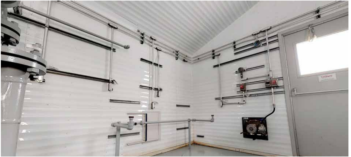
Air Compressors - Pre-wired and spaced for 2 x Instrument Air Compressors
