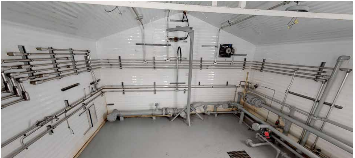
Suction Piping Area: Lots of space to install Charge Pump(s), Skim Pumps, Additional Suction Header Piping - Your choice!
