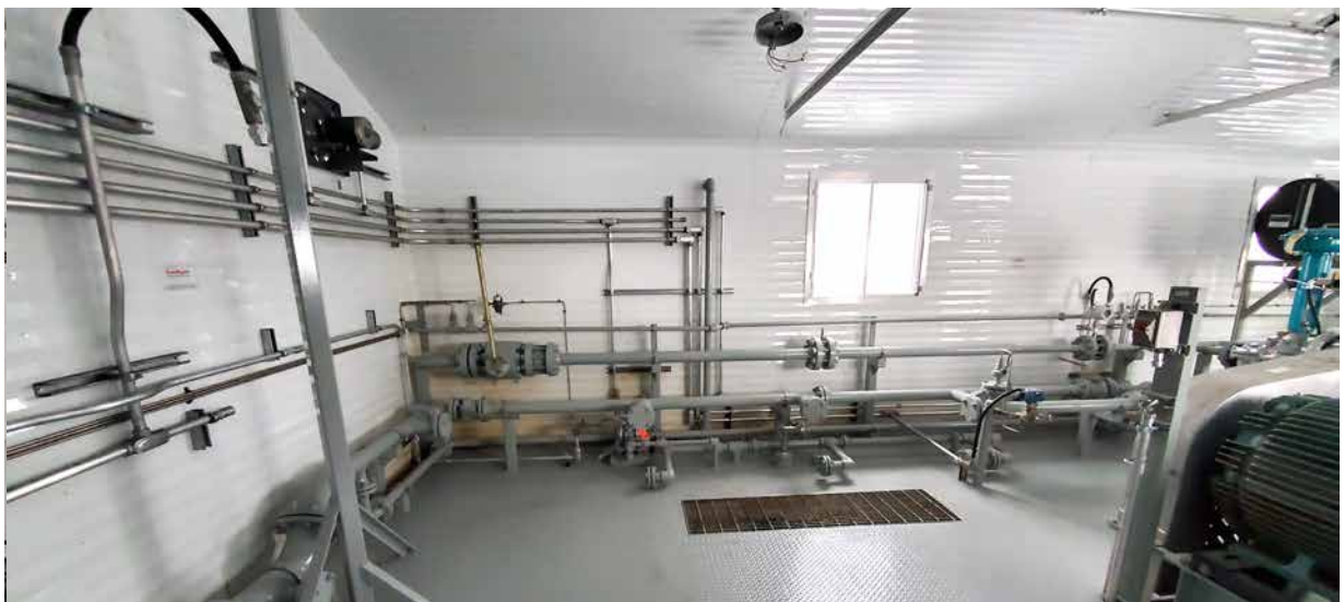
Filter Provisions: Capacity for multiple filter configurations - all draining to sealed sump.
