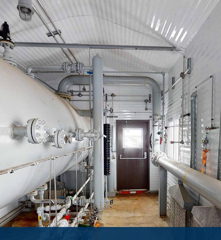
This separator is in great condition – built for sour and only ever used in sweet service. Commissioned in 2008, the vessel is currently setup for 2 phase service (water dump and panic dump), however all the connections and weir exist for it to have a 3rd phase added (1 week delivery and ~\$10,000). Full drawings, over 80 pictures, and more detailed information available upon request! Call us today!
